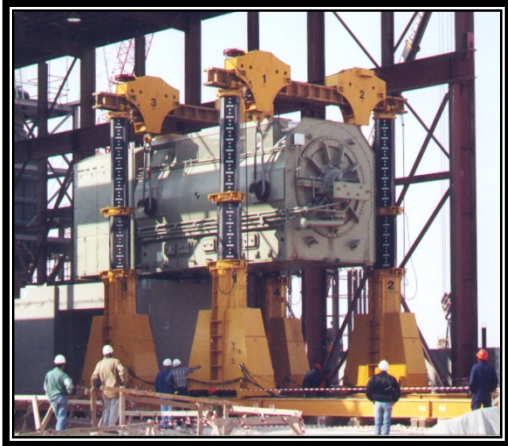
J&R 1402-4-39 Octagon LIFT-N-LOCK Hydraulic Boom Gantry with 150 Ton PowerLinks on a project in Riyadh, Saudi Arabia
