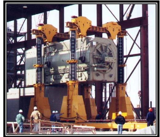
J&R 1402-4-39 Octagon LIFT-N-LOCK Hydraulic Boom Gantry with 150 Ton PowerLinks on a project in Riyadh, Saudia Arabia
